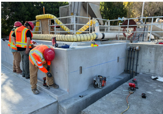
Figure 1 –New Channel at Headworks
