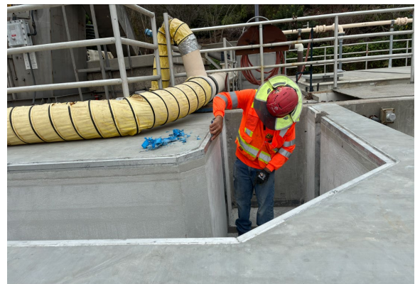
Figure 2 – New Channel at Headworks
