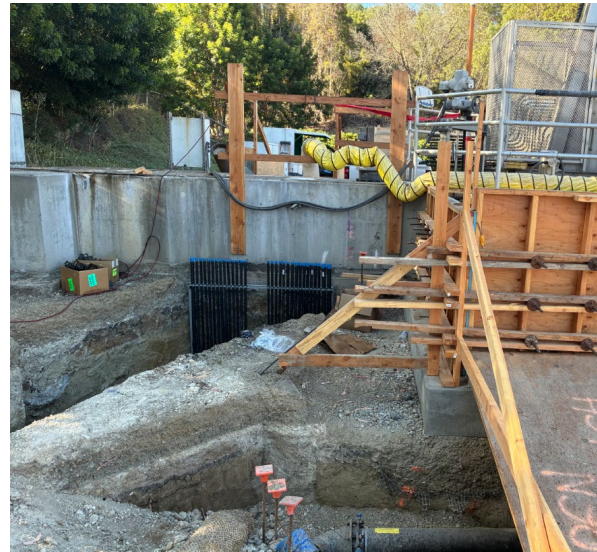
Figure 5 –Forming New Channel at Headworks
