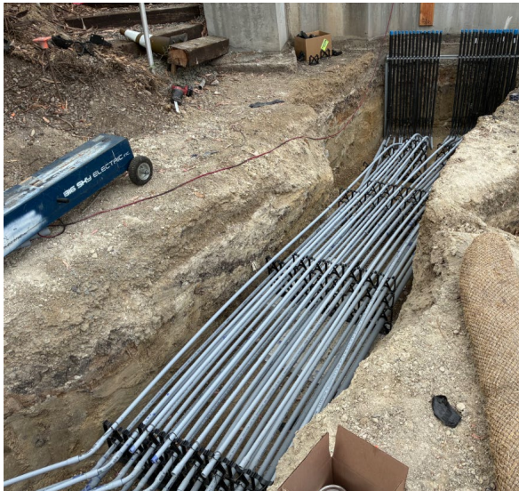
Figure 4 – Routing New Conduit for Headworks Control Panels
