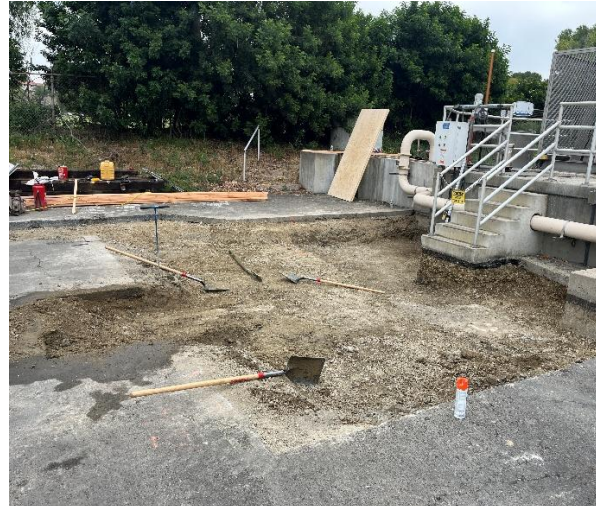
Figure 3 – Excavation at the Headworks
