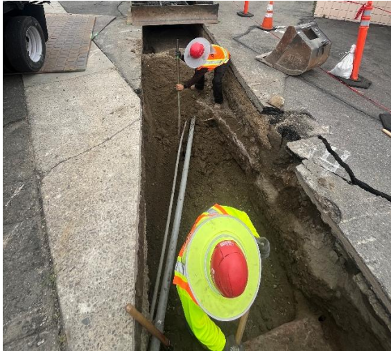
Figure 2 – Yard Piping Excavation
