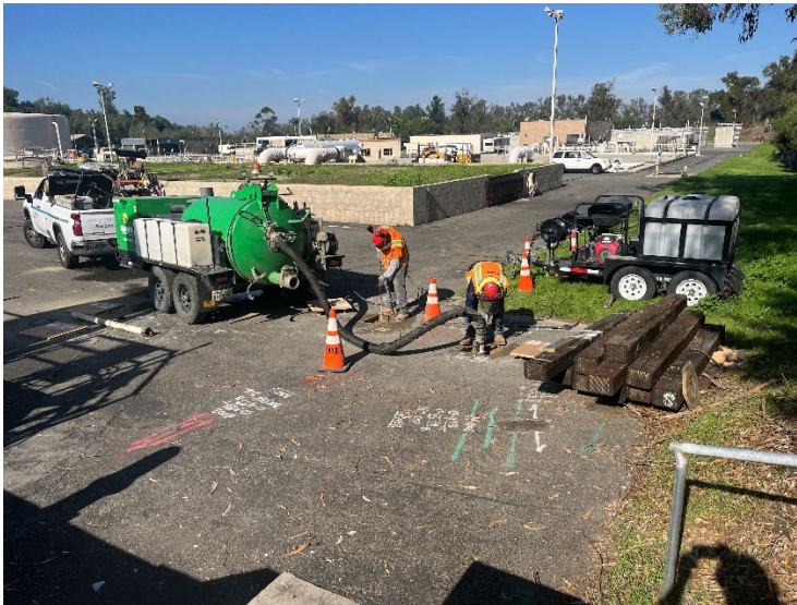
Figure 2 – Potholing at the WRP
