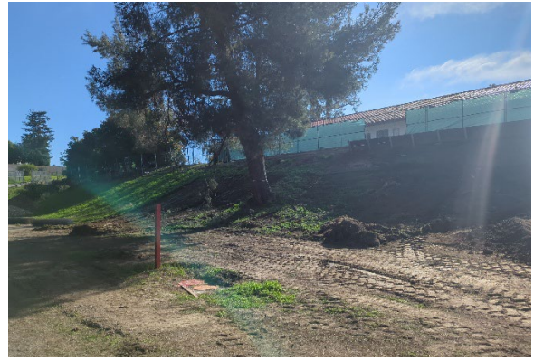
Figure 5 – Temporary Fence Installation
