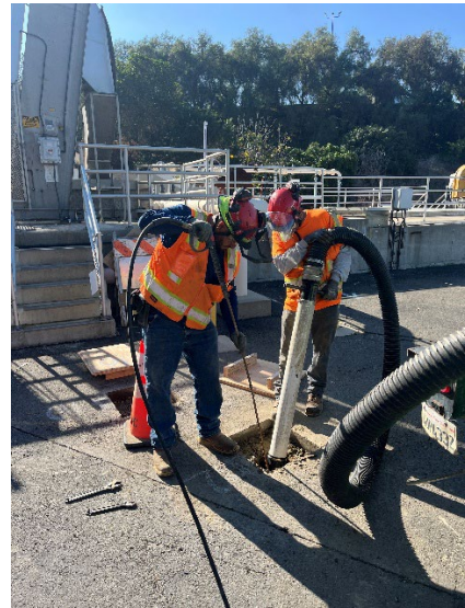
Figure 3 – Potholing at the WRP
