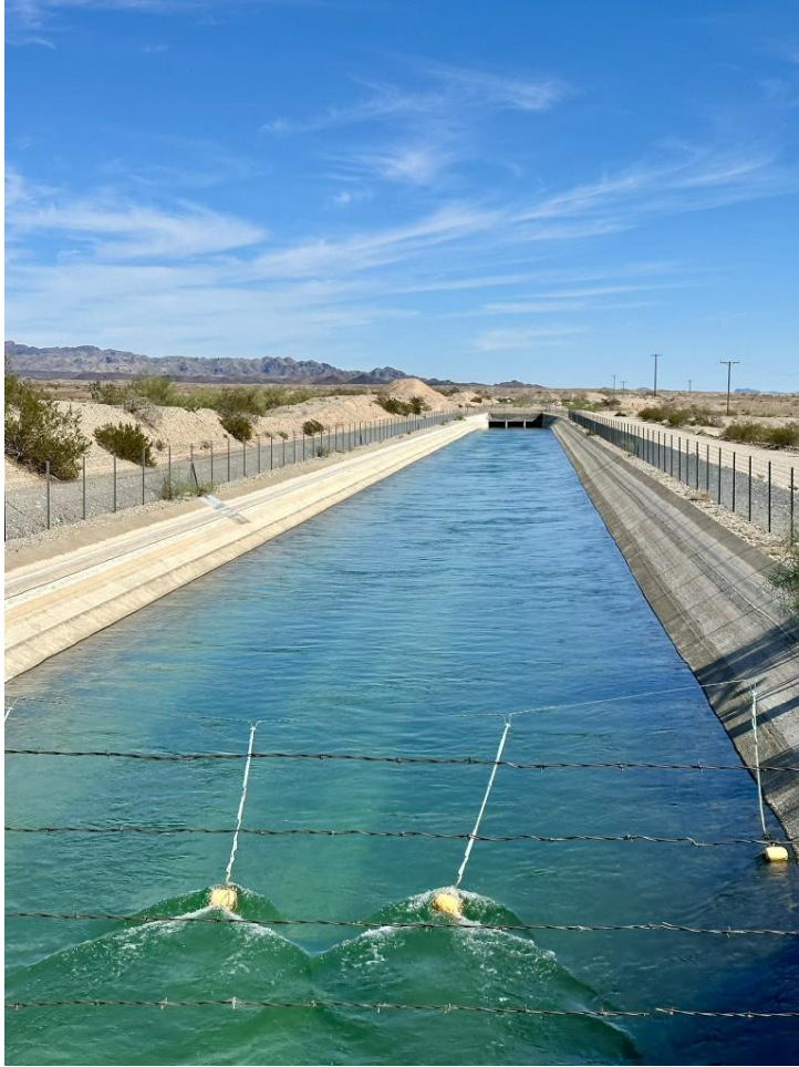
Colorado River Aqueduct
