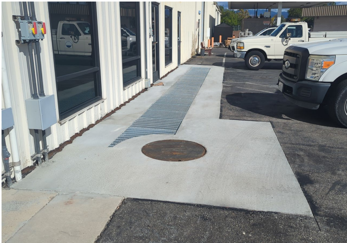
Figure 2 – New Pump Station and Trench Drain
