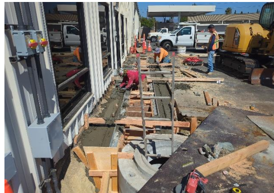
Figure 2 – Trench Drain Concrete Placement
