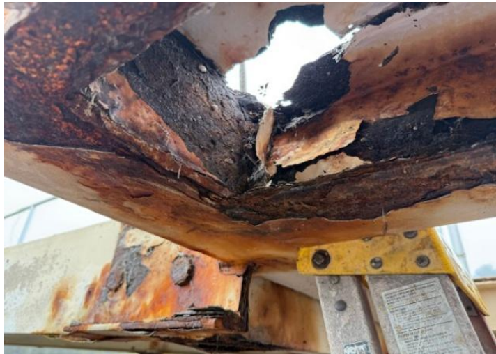
Figure 4 – Corroded Bridge Adaptor Support Beams
