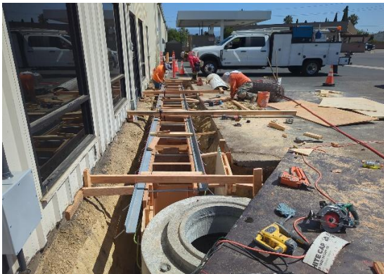
Figure 1 – Trench Drain Formwork
