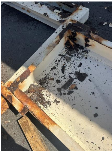
Figure 3 – Corroded Bridge Support Beams
