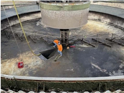
Figure 3 – Dewatered Secondary Clarifier No. 4
