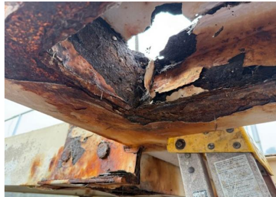
Figure 6 – Corroded Bridge Adaptor
