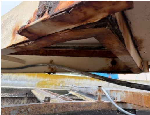
Figure 5 – Corroded Bridge Adaptor
