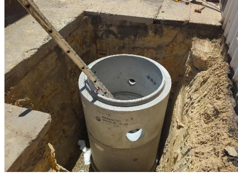
Figure 8 – Precast manhole installation
