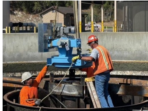
Figure 4 – New Secondary Clarifier No. 4 Drive
