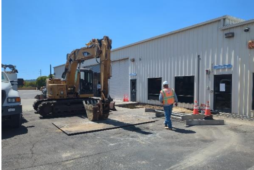
Figure 7 – Precast manhole excavation
