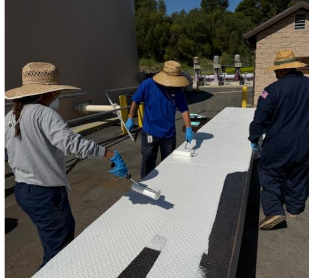
Figure 4 – Priming the Walkway
