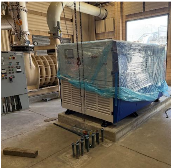
Figure 1 – New Blower Placement
