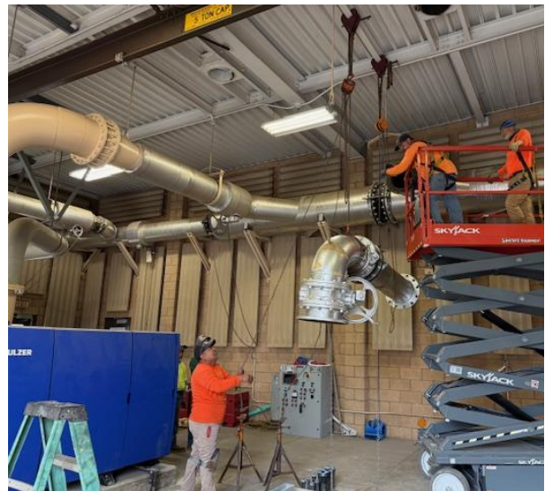
Figure 2 – Suction Piping Reconfiguration
