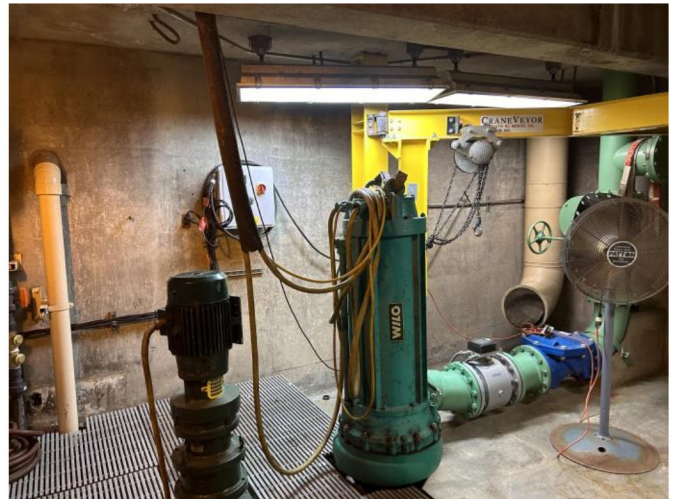
Photograph 16. Lower subterranean level of ACLS with grate over suction pipe, gate valve, grinder, and motor at left and check valve at right background, camera facing east
