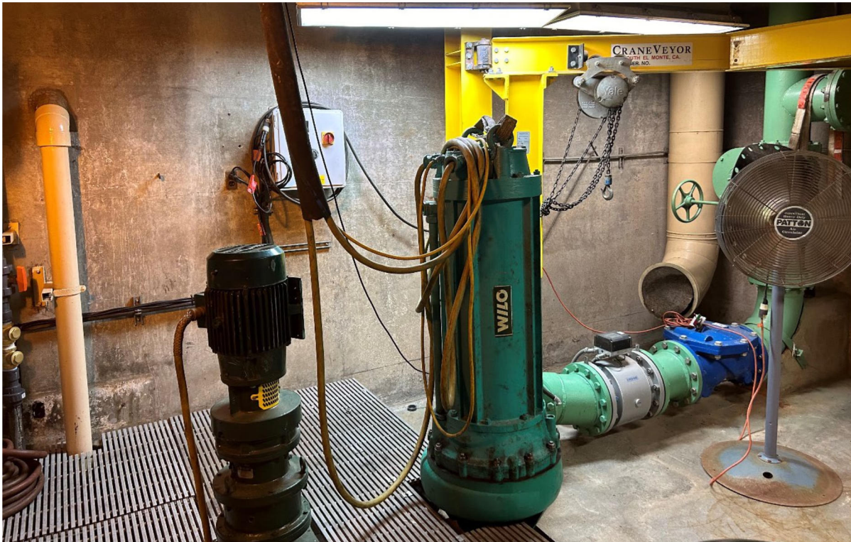
Photograph 12 View of Lower Subterranean Level of ACLS, with Grate over Suction Pipe, Gate Valve, Grinder, and Motor (Left) and Check Valve (Background Right), Facing East
