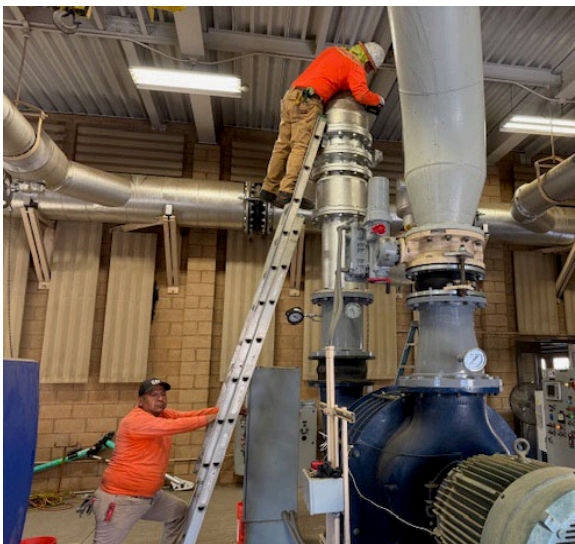
Figure 1 – Disconnecting Suction Piping
