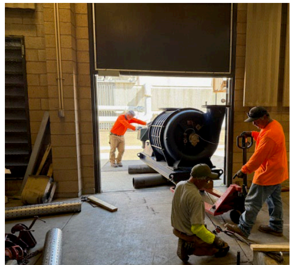
Figure 2 – Removing Existing Blower
