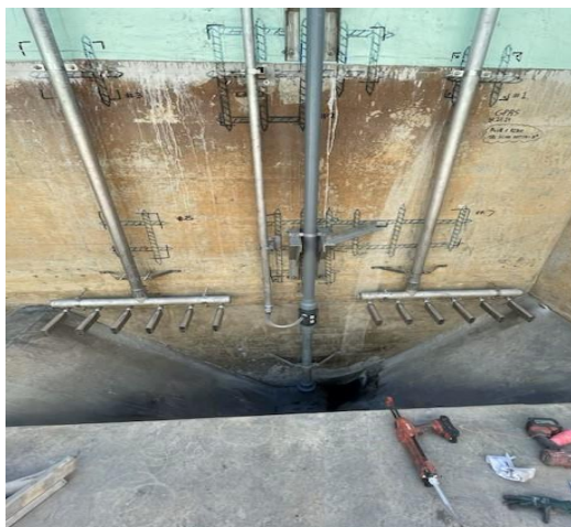
Figure 1 – New Mechanical Piping and Diffusers
