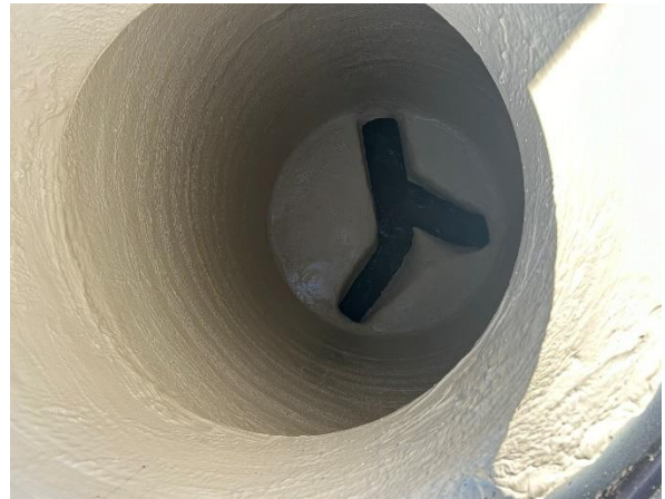
Figure 9 – New Lining in Manhole
