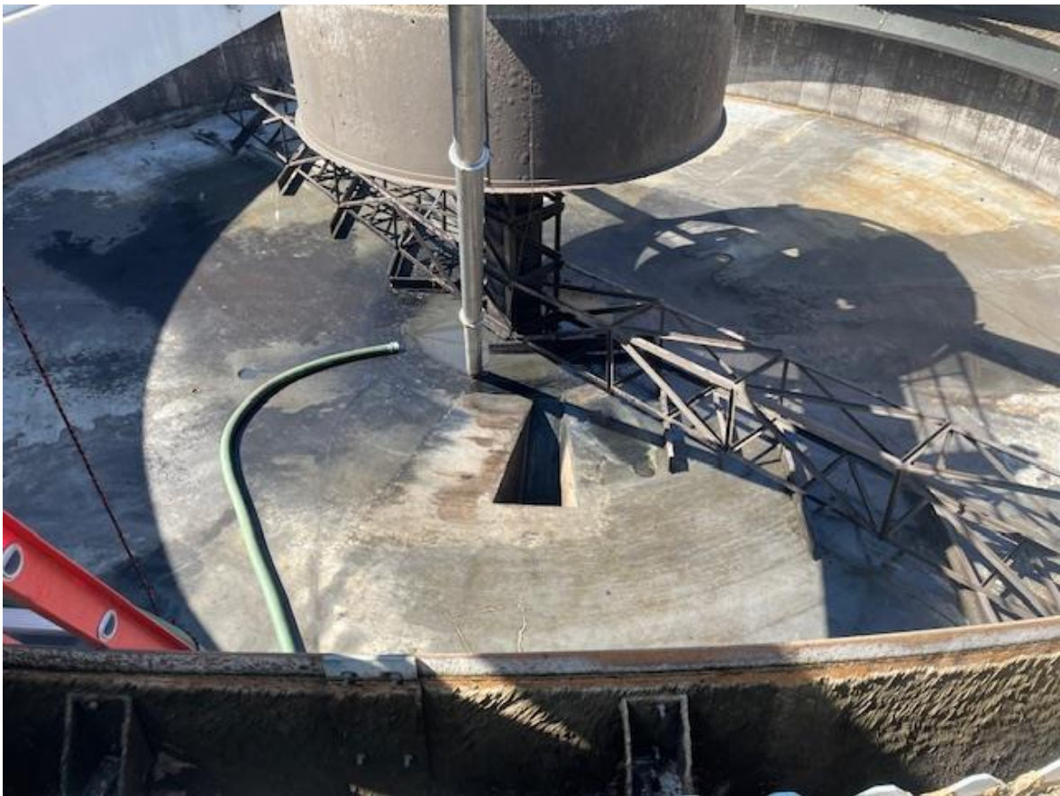
Figure 7 – Dewatered Secondary Clarifier No. 3
