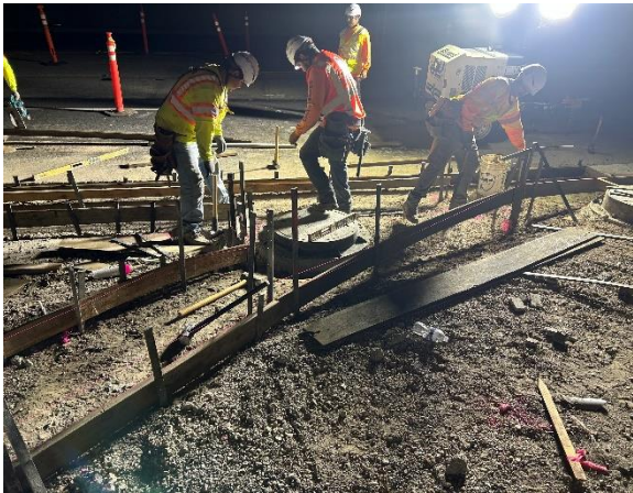
Figure 8 – Regrading around Manhole
