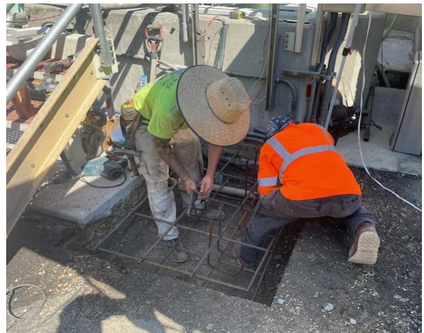
Figure 2 – Rebar Placement for PLC Pad
