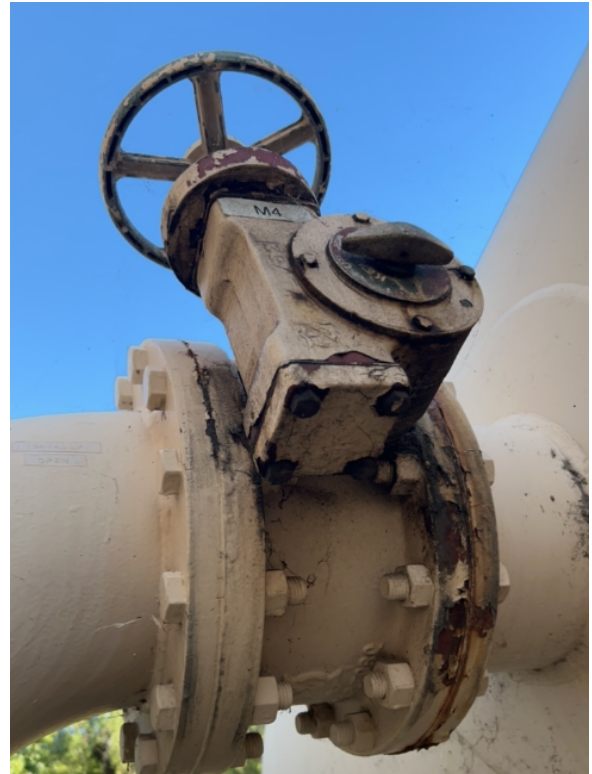
Figure 6 – OOPS Surge Tank Isolation Valve
