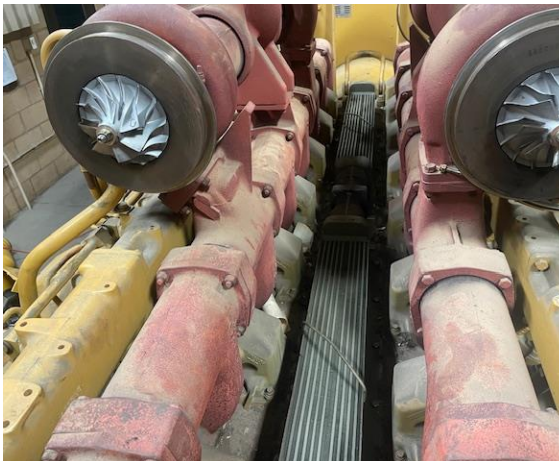
Figure 7 – Inner Cooler Rehabilitation
