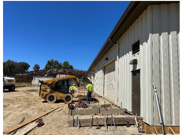
Figure 4 – Exterior Formwork
