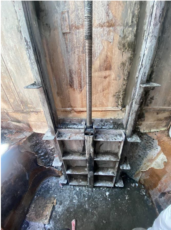
Figure 3 – Northline Inlet Gate before Coating Repair
