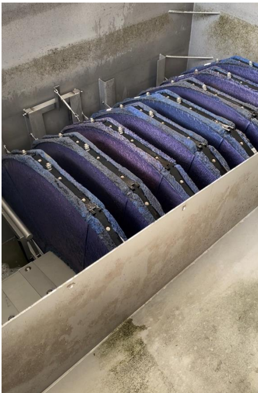
Figure 1 - Existing Tertiary Filter Disks
