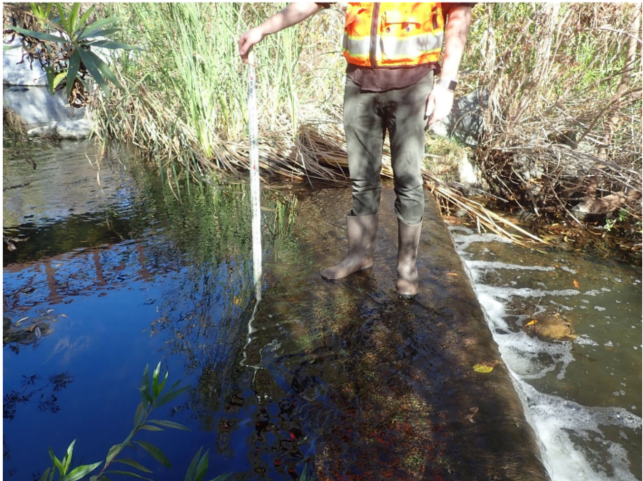
Figure 1 – Exposed ETM Concrete Encasement in Aliso Creek
