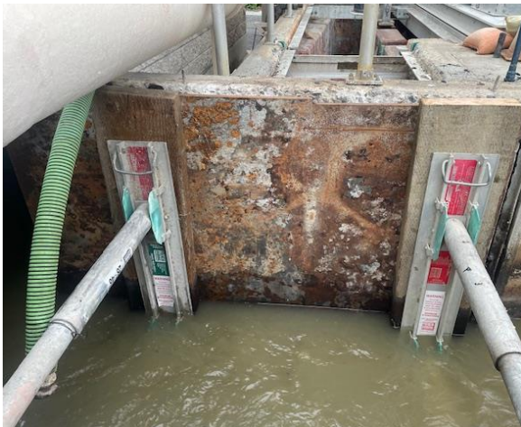
Figure 1 – Cofferdam Installation
