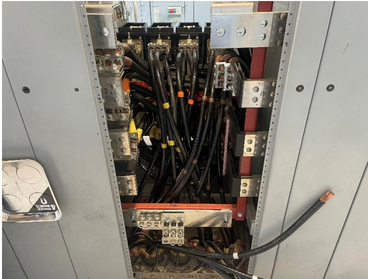
Figure 3 – New ATS in the WRP Main Electrical Room
