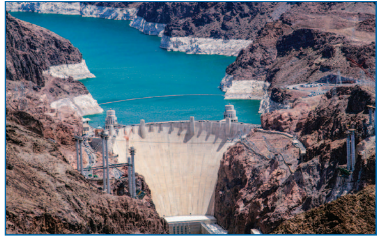
Hoover Dam, on the Colorado River (Lake Mead behind it).
