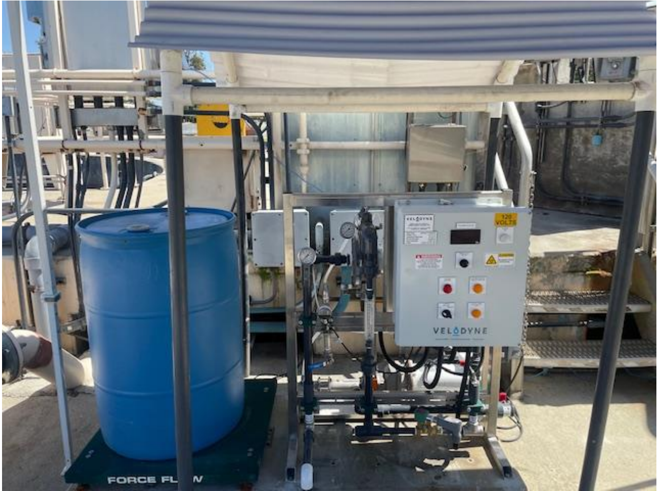
Figure 4 – Polymer Test Skid installed at WRP
