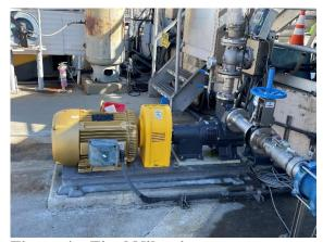
Figure 4 – Final Nikuni pump installation.
