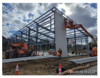
Figure 2 – PEMB Installation
