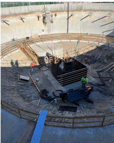
Center column foundation replacement for a circular clarifier.
