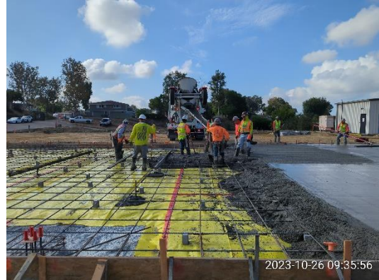
Figure 3 – New Warehouse Slab
