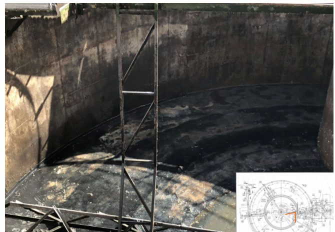
Figure 2 – Drained Secondary Clarifier
