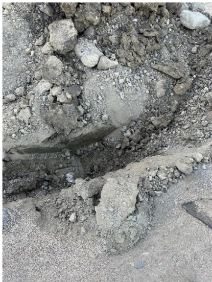
Figure 1 – Moist Subgrade Conditions
