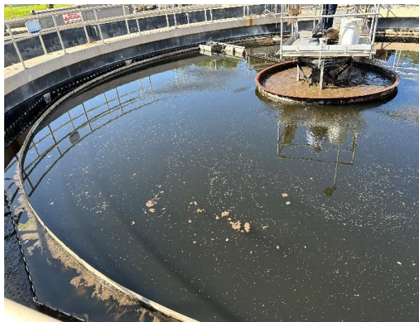
Figure 1 –Secondary Clarifier No. 1
