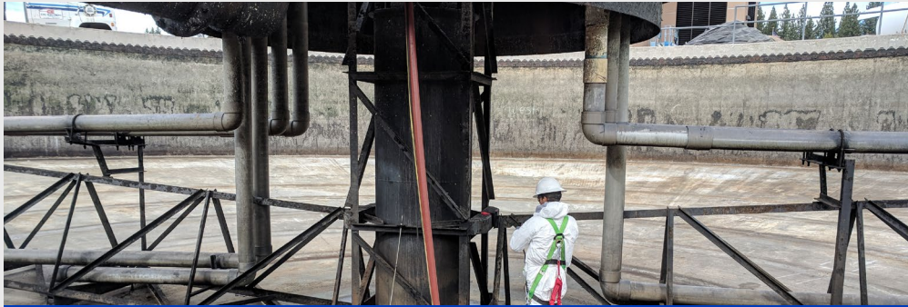
Existing clarifier mechanism with mid-level RAS pipe drawoff.
