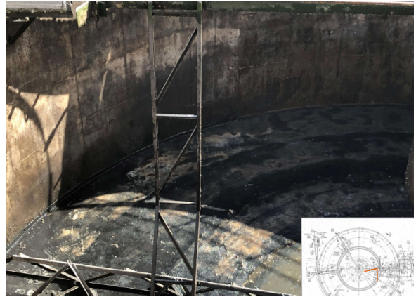
Figure 3 – Drained Secondary Clarifier
