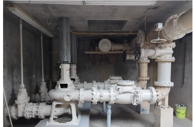
Figure 7 – New Effluent Pumps
