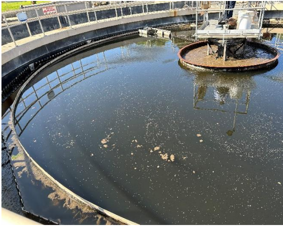
Figure 2 –Secondary Clarifier No. 1
