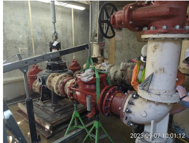
Figure 6 – New Effluent Pump No. 2
