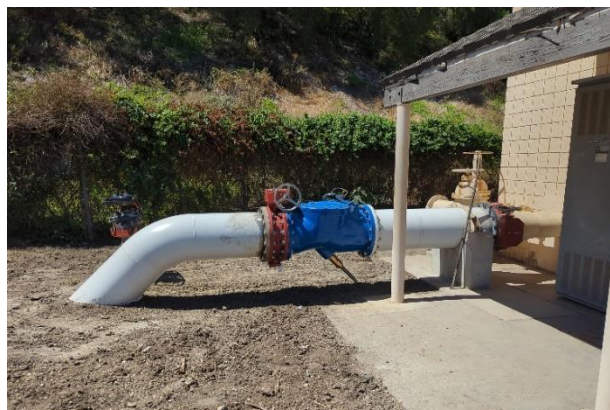
Figure 5 – Effluent Transmission Main Check Valve Installation
