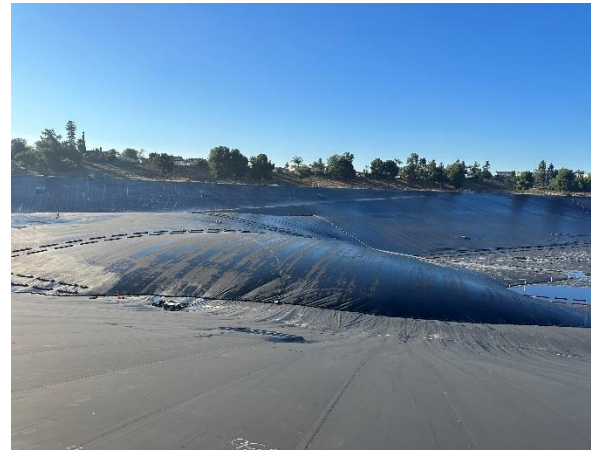
Figure 2 – Floating Cover Inflation
