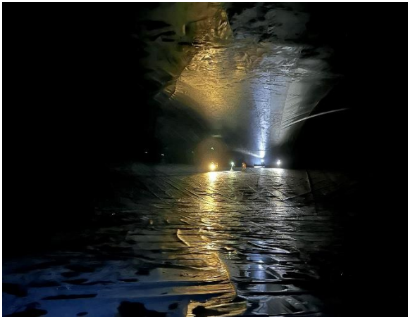
Figure 1 – Floating Cover Inflation
