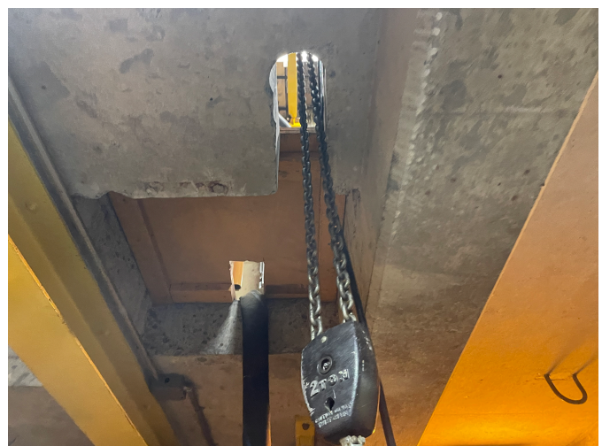
Figure 4. Existing Lifting Line for Pumps
