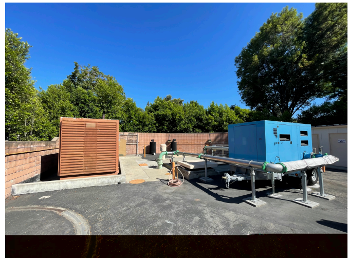
Figure 3. ETWD ACLS generator, trailer mounted emergency standby pump and piping, and wet well/drywell (Below grade)
