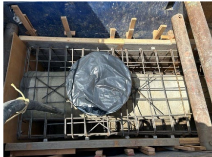
OC Feeder Shutdown – Concrete formwork for access way encasement
