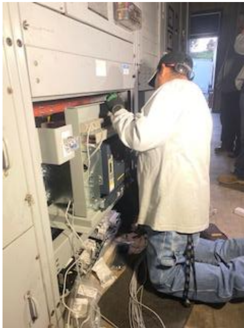
Figure 10 – Breaker Installation in the Main Electrical Room
