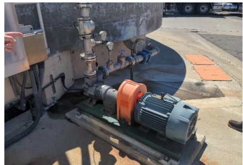
Figure 1 – Existing DAF Unit 2 Nikuni Pump
