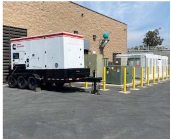
Figure 13 – Portable Generator at Main Electrical Building
