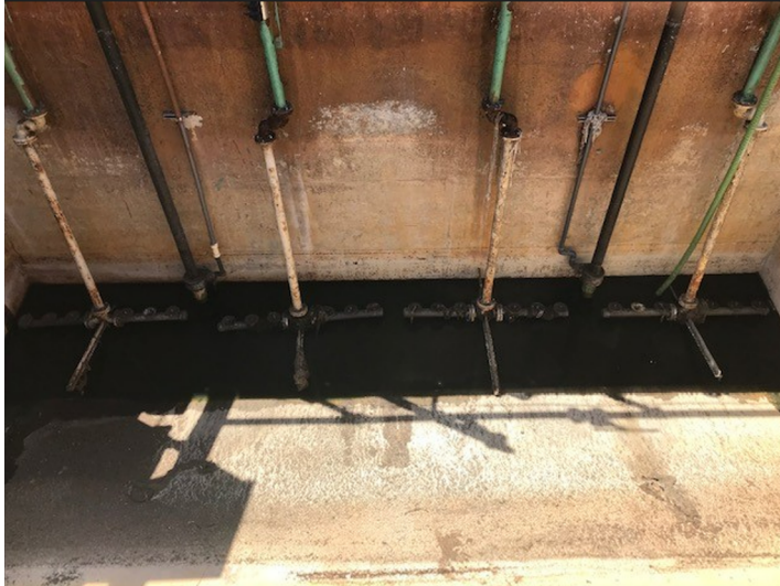
Figure 1 – Current Grit Aeration Diffusers
