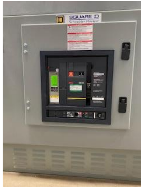
Figure 11 – New 4,000 amp Breaker
