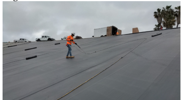
Figure 4 – Air Lance Testing
