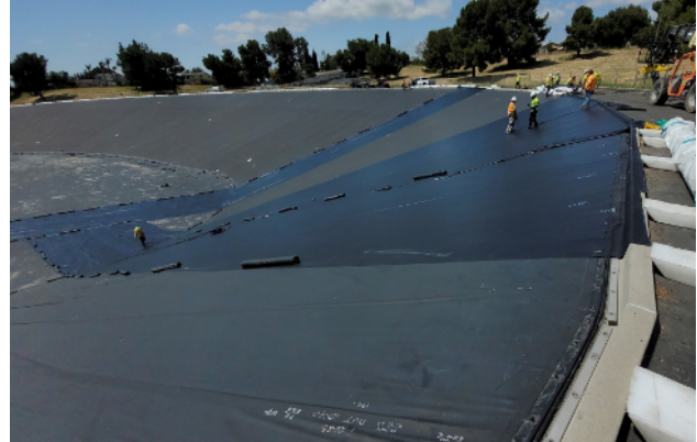
Figure 6 – Floating Cover Installation on Bench
