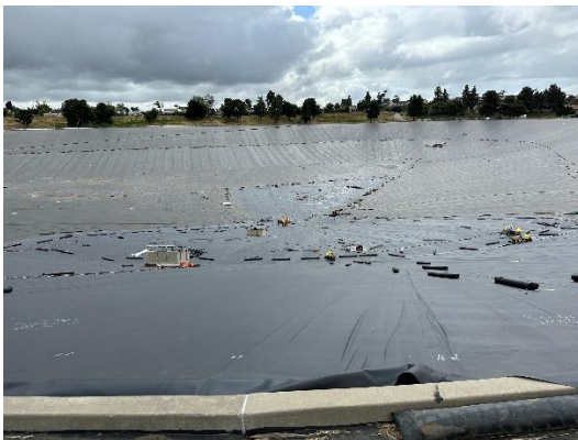
Figure 1 – Final Liner Installation
