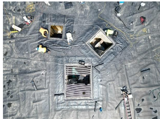
Figure 2 – Liner Installation around Vaults
