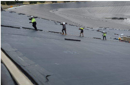
Figure 3 – Sand Tube Placement
