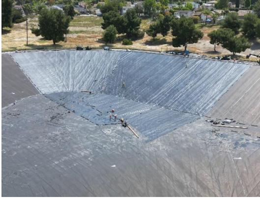
Figure 5 – Drone Footage of Floating Cover Installation on Bench
