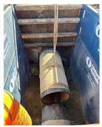
OC Feeder Shutdown - Access Point for Liner Replacement
