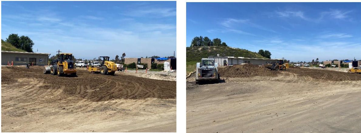
Figure 3 - Filter Plant Backfill
