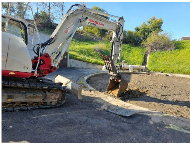
Figure 4 – Clearwell Curb Demolition
