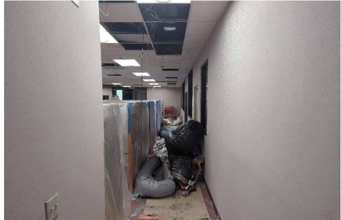
Figure 6 – Main Office Duct Replacement
