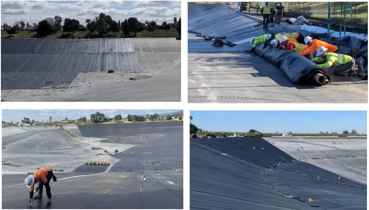
Figure 1 - Liner Installation
