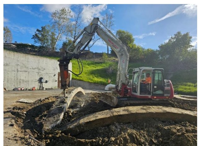
Figure 4 – Clearwell Curb Demolition
