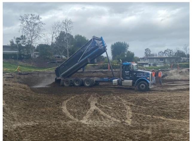
Figure 3 - Filter Plant Backfill
