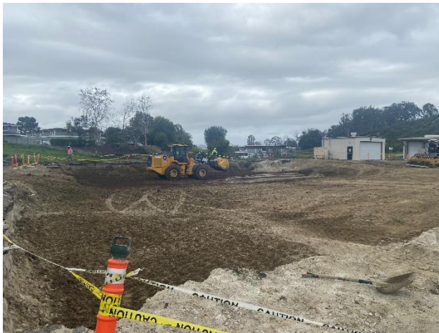
Figure 3 - Filter Plant Backfill
