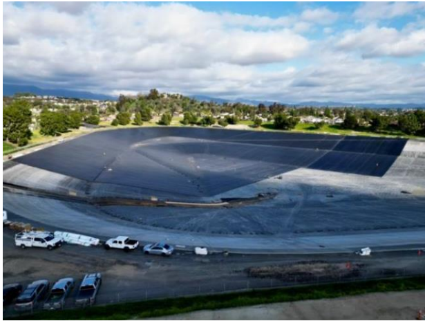
Figure 2 - Liner Installation
