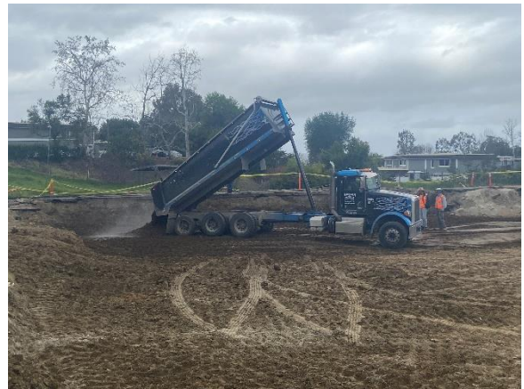
Figure 4 – Backfill Import Material
