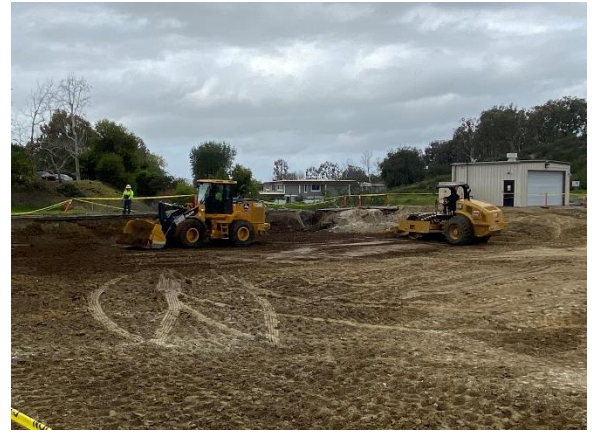
Figure 6 – Backfill Operations
