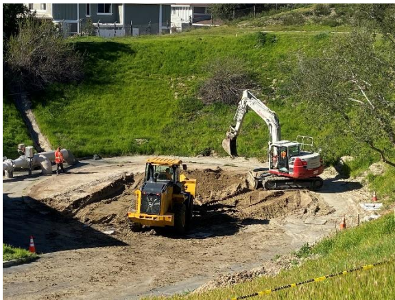
Figure 3 – Clearwell Sand Removal
