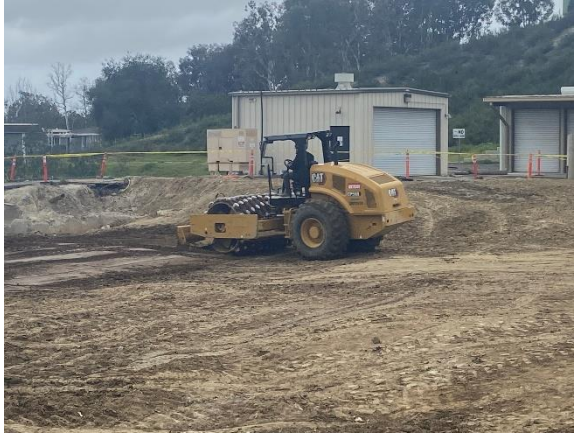
Figure 5 – Backfill Compaction
