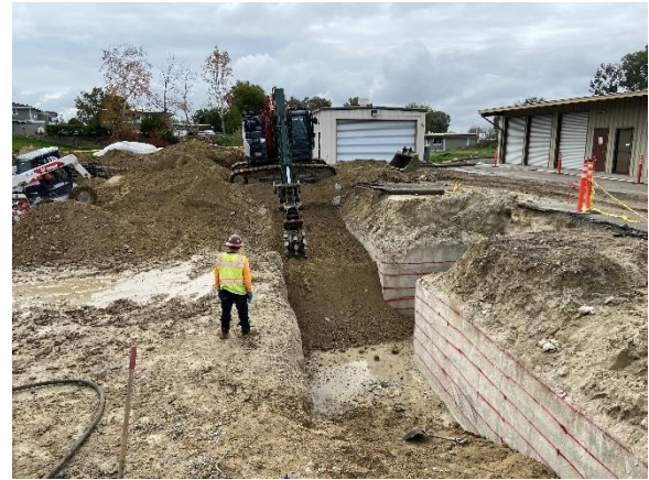
Figure 4 - Vault Backfill
