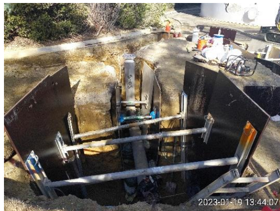
Figure 6 – Underground Piping
