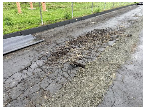
Figure 1 Perimeter Road Paving Deterioration
