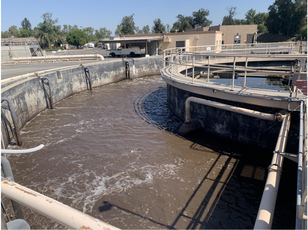
Figure 1 – Secondary Clarifier No. 1 surrounded by the WAC
