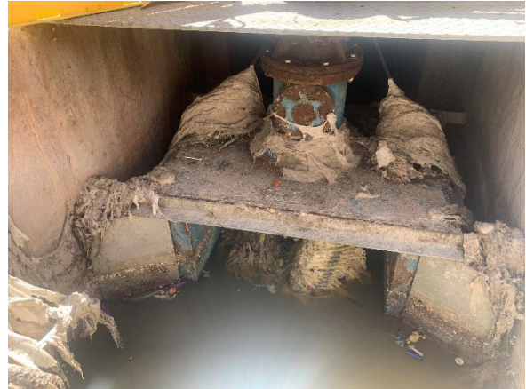
Figure 2 – Bypass Channel Dimminutor
