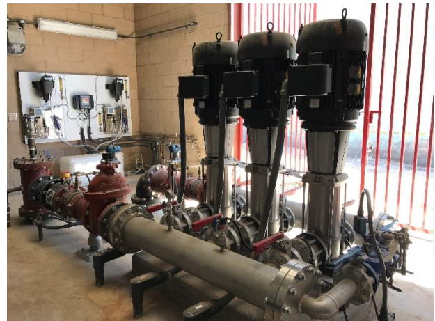
Figure 2. Skid-Mounted Packaged Booster Pump Station (1,100 gpm) at Morrow Hills Pump Station
