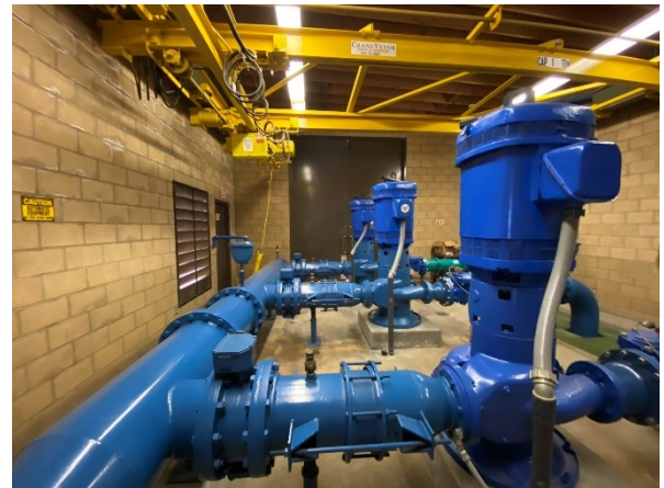
Figure 1. ETWD PS-1 Vertical Single-Stage Split Case Pumps, Bridge Crane, and Double Leaf Access Doors
