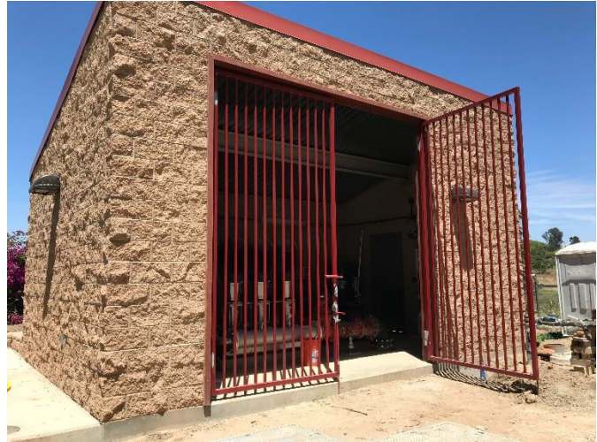
Figure 3. Morrow Hills Pump Station CMU Building and Double Leaf Gate Access Opening (Site Pavement Not Yet Constructed)
