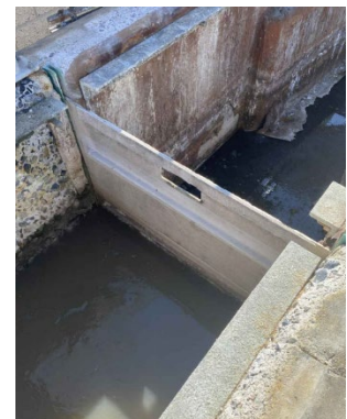
Figure 2 – Grit Chamber Inlet Isolation Gate
