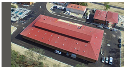
Baker Water Treatment Plant
