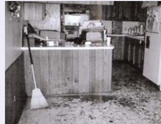
Excessive amounts of fats, oil and grease in the private sewers can result in raw sewage overflowing into your home.
