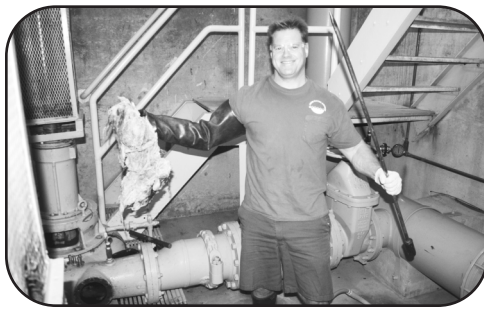
ETWD employee, Stuart Kain, removing debris from a sanitation pump.
