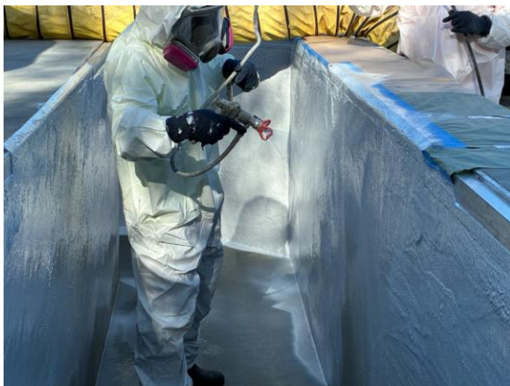
Figure 1 –Coating the New Channel at Headworks
