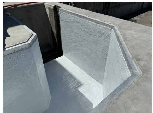
Figure 2 – Coated New Channel at Headworks
