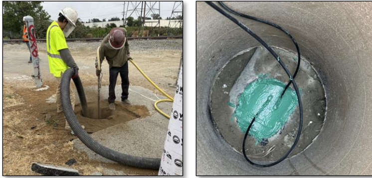
Figure 12 – Typical Potholing Activities
