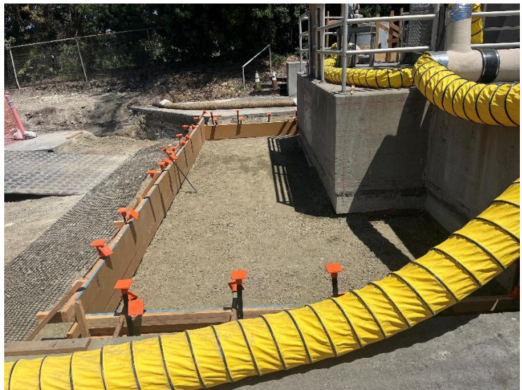
Figure 2 – Concrete subgrade formwork at the Headworks
