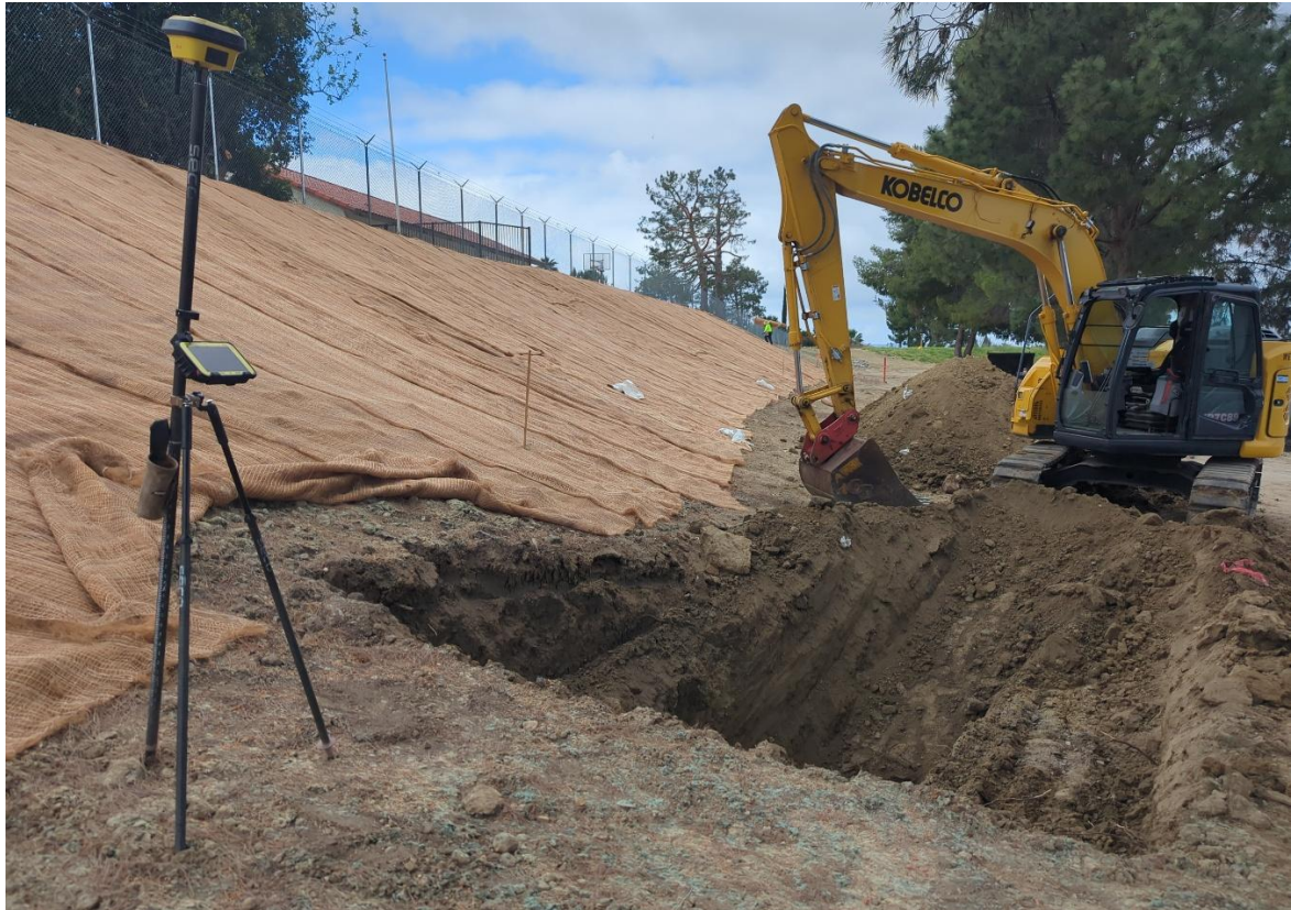
Figure 1 – Slope Landscaping and Hydrant Relocation
