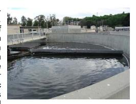
The project replaces and up-dates the Clarifier Nos. 3 and 4 scum station with a more efficient, lower maintenance and more flexible system. The project installs a self-contained package lift station system that will allow the skimmed scum to gravity flow into a wet with submersible pumps controlled by a float system. The project will improve the operation and reliability of the clarifiers and replace the existing obsolete equipment.
