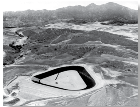
1967 construction of the uncovered 233-million-gallon R-6 Reservoir enabled the El Toro Water District to store imported water for later use.
