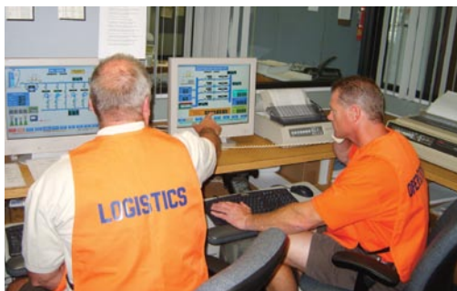
Centralized System Monitoring
