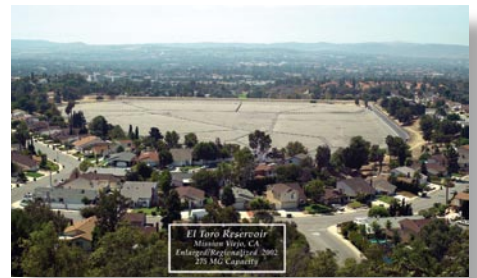
R-6 Reservoir expanded and covered in 2002.
