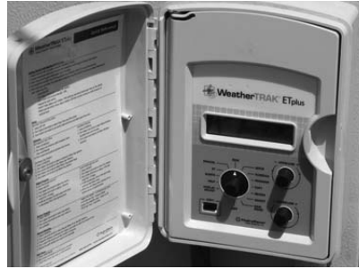
Photo of ETWD's new Smartimer Control box in the their new California Friendly and Native Plant Garden.
